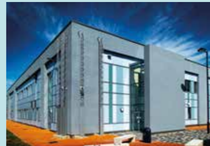
■ Parkway – Advanced Engineering Centre
